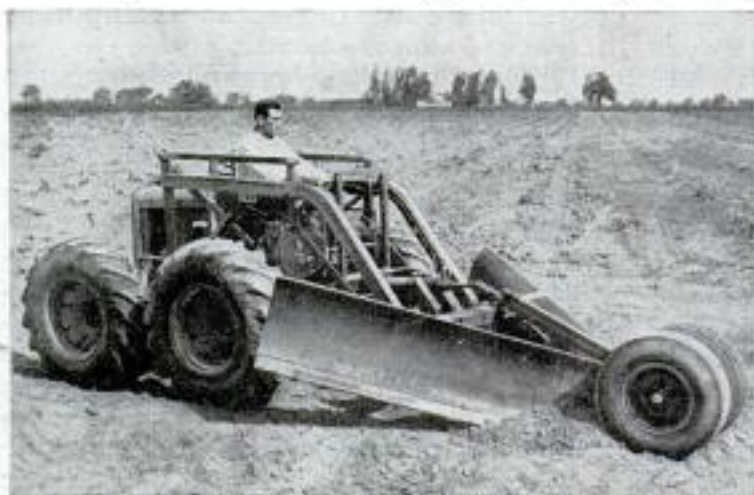
Another home-built machine is a hydraulic fork lift that will raise 1000 pounds to height of nine feet. Here it is used to move beehives to alfalfa field. Below, home-designed ditcher has two hydraulic controls to raise, lower and tip the blade
